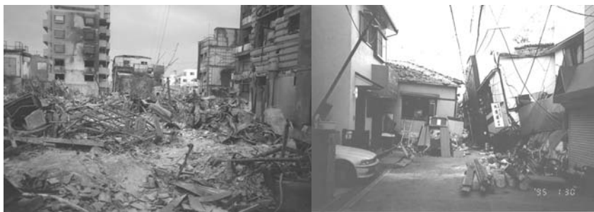
Fig.6.1. The Great Hanshin-Awaji Earthquake Disaster. Inner city
