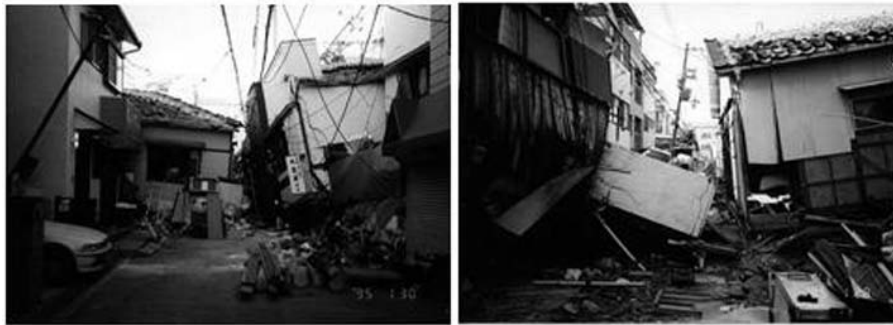
Fig.6.3. Street blockade caused by housing collapse
