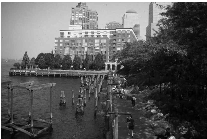
Figure 13.2 Battery Park City, New York. Innovative public spaces and infrastructure were installed by the public development corporation in advance of development, setting the tone for the development. Source: Gary Hack.
