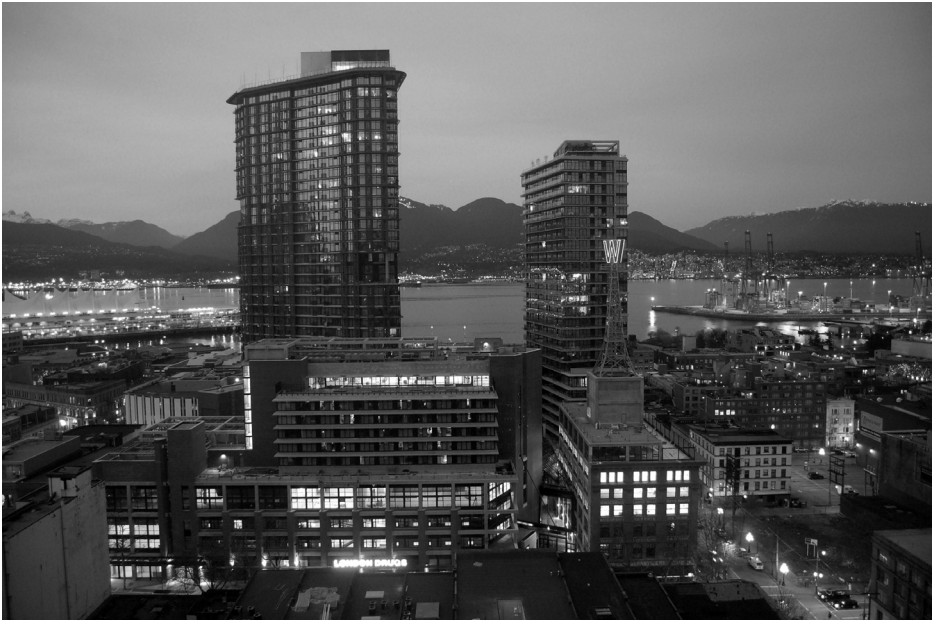
Figure 13.8 Woodward Development, Vancouver. A complex mixed use development was made possible in part by allowing greater heights and densities than are normally permitted. Reproduced by permission of Henriquez Partners Architects.
